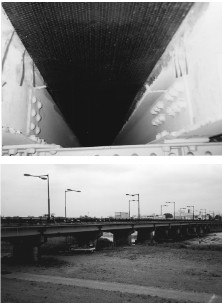
Fig. 8.19—Overview of bridge rehabilitation with Forca Tow Sheet, Japan
