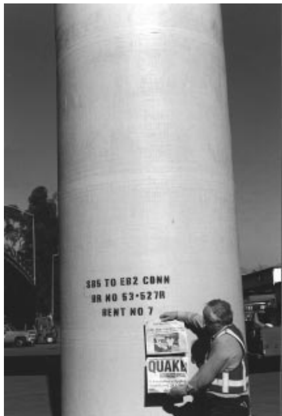
Fig. 8.14—Bridge column wrapped with GFRP, California
