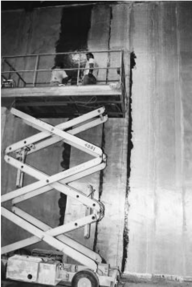
Fig. 8.17—Repair and strengthening of tilt-up concrete walls damaged during the 1994 Northridge earthquake
